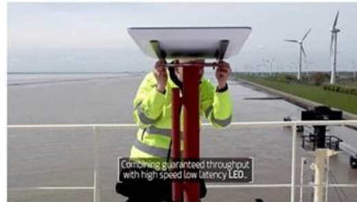
Installation of Starlink (youtube)
