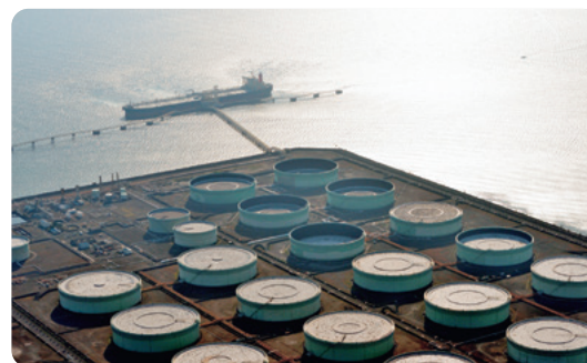
Crude oil storage tanks with a tanker in the background
